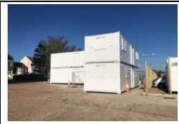
25th October - site offices and welfare in place
