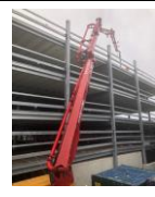
19th November - first day of the concrete pour to the decks
