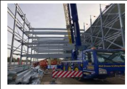
23rd October - final series of beams being installed
