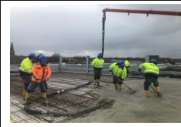
19th November - concrete pour to the top deck
