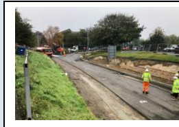
15th October - base course being laid in Dover Street
