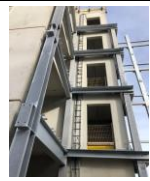
23rd October - first fix electrics to stair cores and lift shafts
