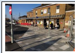
11th December - paving complete leading to station entrance
