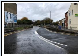
7th November - Dover Street complete and ready for opening
