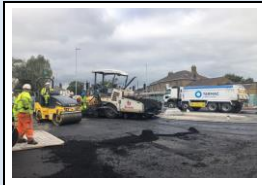
3rd October - surface course to the new roundabout
