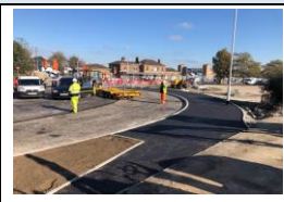
25th October - new footway constructed in Dover Street
