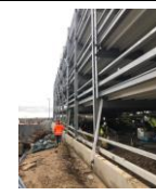
6th December - installation of rainwater downpipes
