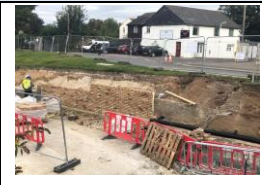
3rd October - Construction of the new retaining wall in Dover Street
