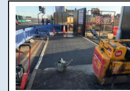
11th December - construction of the commercial crossover for the site exit
