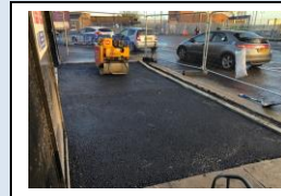
30th November - construction of the commercial crossover for the site entrance
