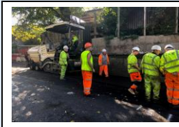
11th October - surface course being laid to Milton Road
