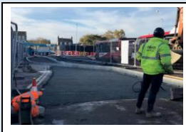
8th November - granular base course being installed in the bus terminus
