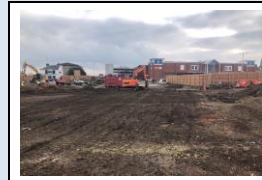
21st November - preparation of the piling mat
