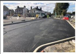
1st October - surface course laid to the taxi rank area
