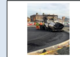
23rd October - base course being laid in Dover Street
