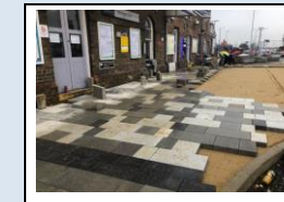
26th November - paving to the station frontage
