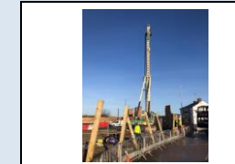
18th December - commencement of the CFA piling on site
