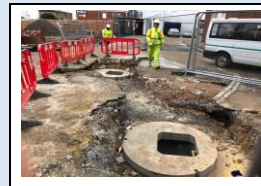
19th November - additional drainage being installed in Station Street
