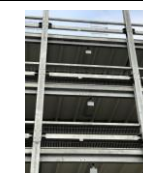
3rd January - anti-climb mesh being installed
