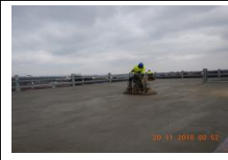
20th November - power floating the concrete on the top deck
